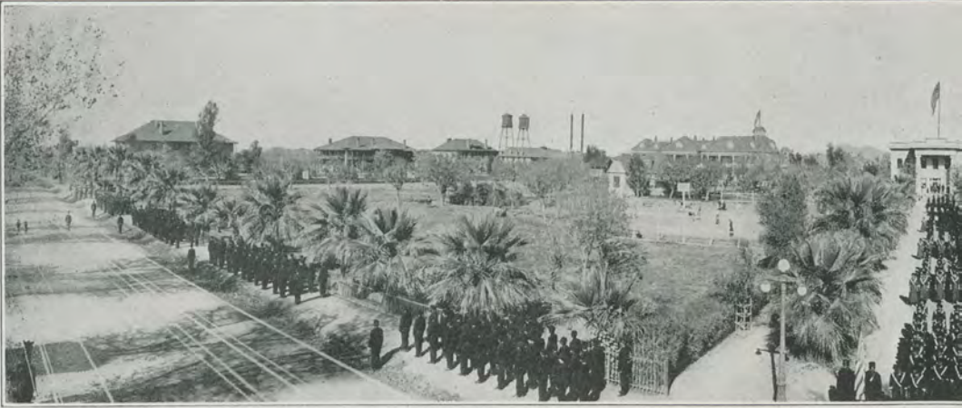
PANORAMIC VIEW OF THE BUILDINGS AND G
