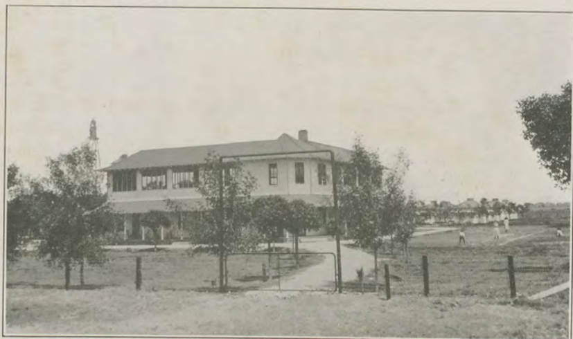
Main Building of the Phoenix Sanatorium
