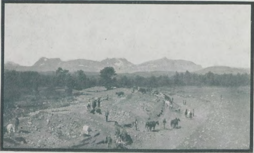
BLACKFEET INDIANS AT WORK ON THE CUTBANK CANAL ON THEIR RESERVATION IN MONTANA BUILT BY THEM UNDER THE DIRECTION OF U. S. IRRIGATION ENGINEERS
