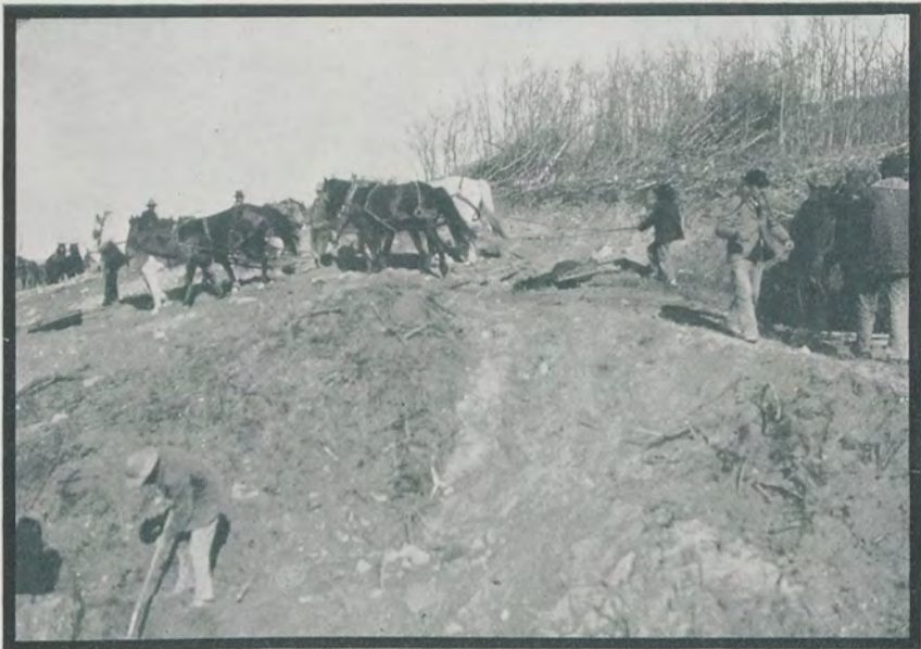
BLACKFEET AT WORK ON THE ST. MARY CANAL—BUILT UNDER THE DIRECTION OF THE UNITED STATES RECLAMATION SERVICE
