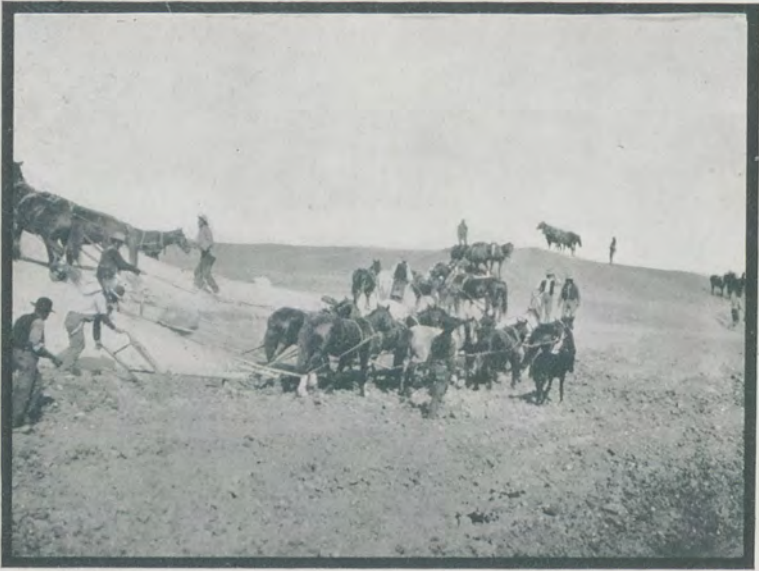
BLACKFEET INDIANS AT WORK ON ST. MARY PROJECT, ALONG THE INTERNATIONAL BORDER BETWEEN UNITED STATES AND CANADA
