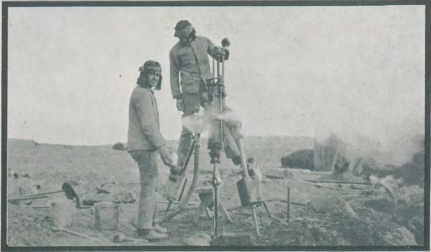
☐ FULLBLOOD NAVAJO INDIANS OPERATING STEAM DRILL ON THE CONSTRUCTION OF THE ZUNI DAM, BLACKROCK, NEW MEXICO
