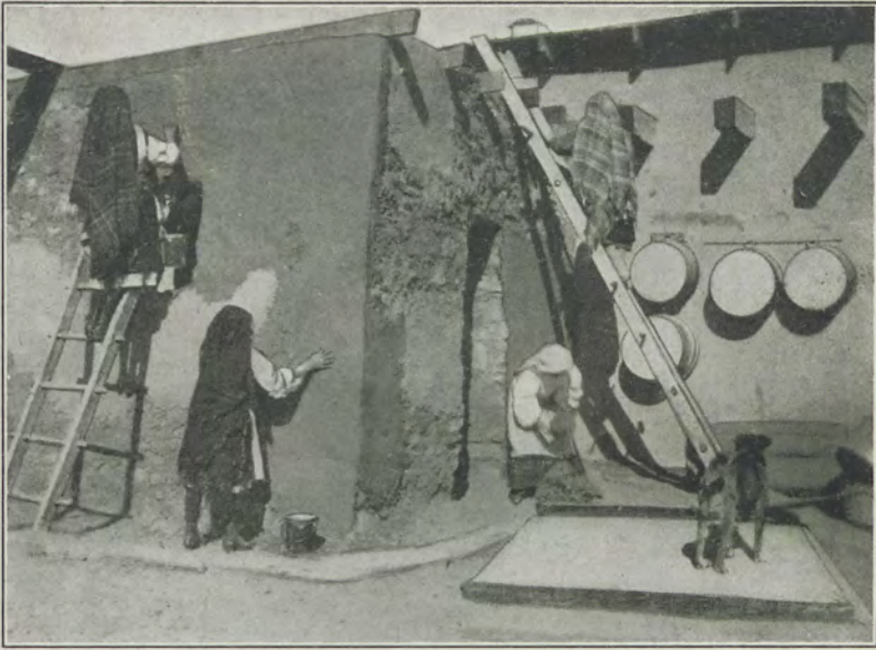
MOTHERS OF PUEBLO CHILDREN ATTENDING THE DAY SCHOOL AT PAQUATE, N. M., PLASTERING THE BUILDINGS
