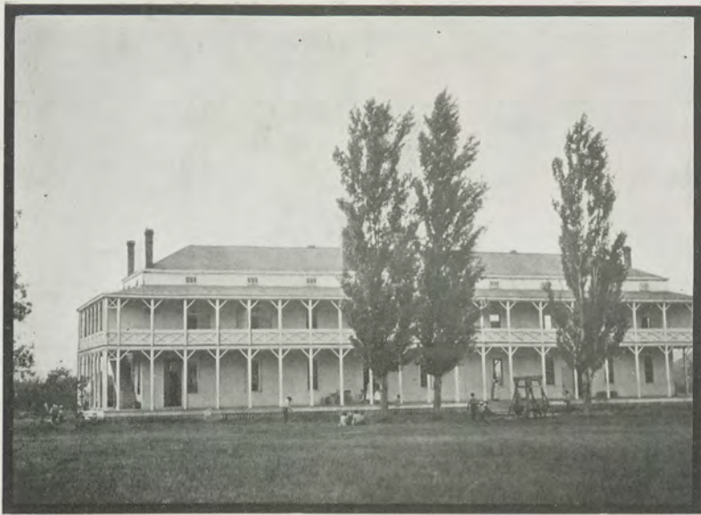
FORT LAPWAI TUBERCULOSIS SANITARIUM SCHOOL—FORMERLY THE POST HOSPITAL AT FORT LAPWAI. CAPACITY, FIFTY STUDENTS
