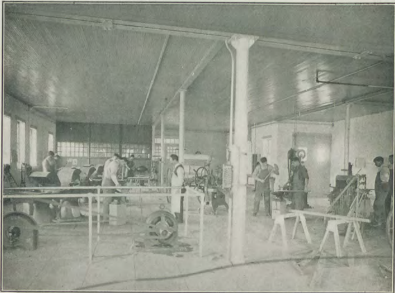
VIEW IN THE BLACKSMITH SHOP
