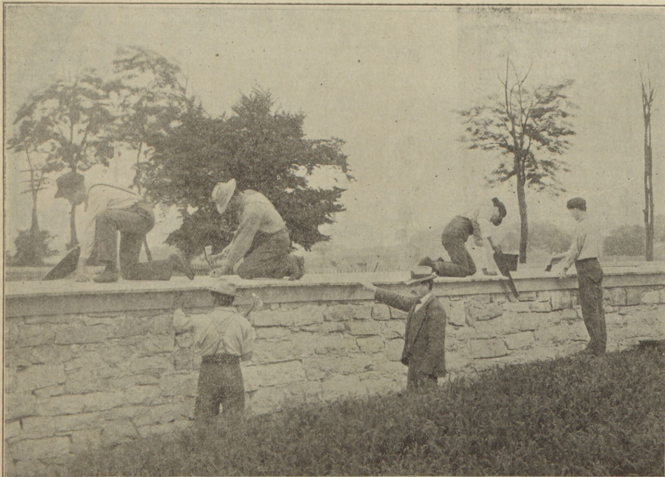
CARPENTER GARDNER AND HIS INDIAN BOYS COPING THE STONE FENCES ON OUR SCHOOL FARM.
