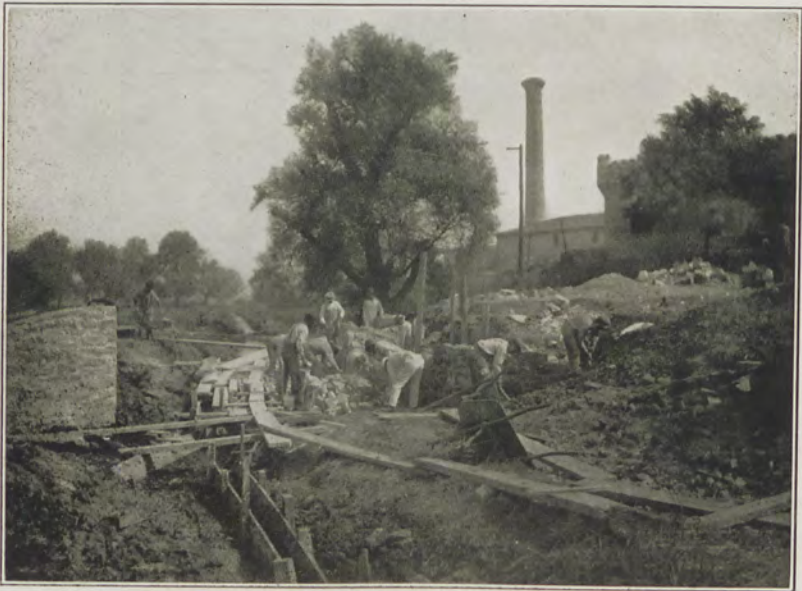
STUDENTS BUILDING STONE BRIDGE ON SCHOOL PROPERTY
