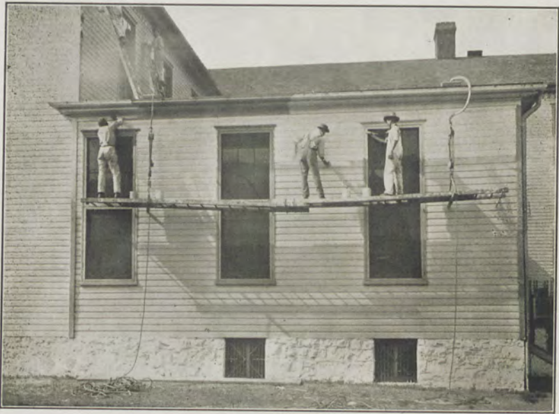
STUDENTS AT WORK REPAINTING DINING HALL
