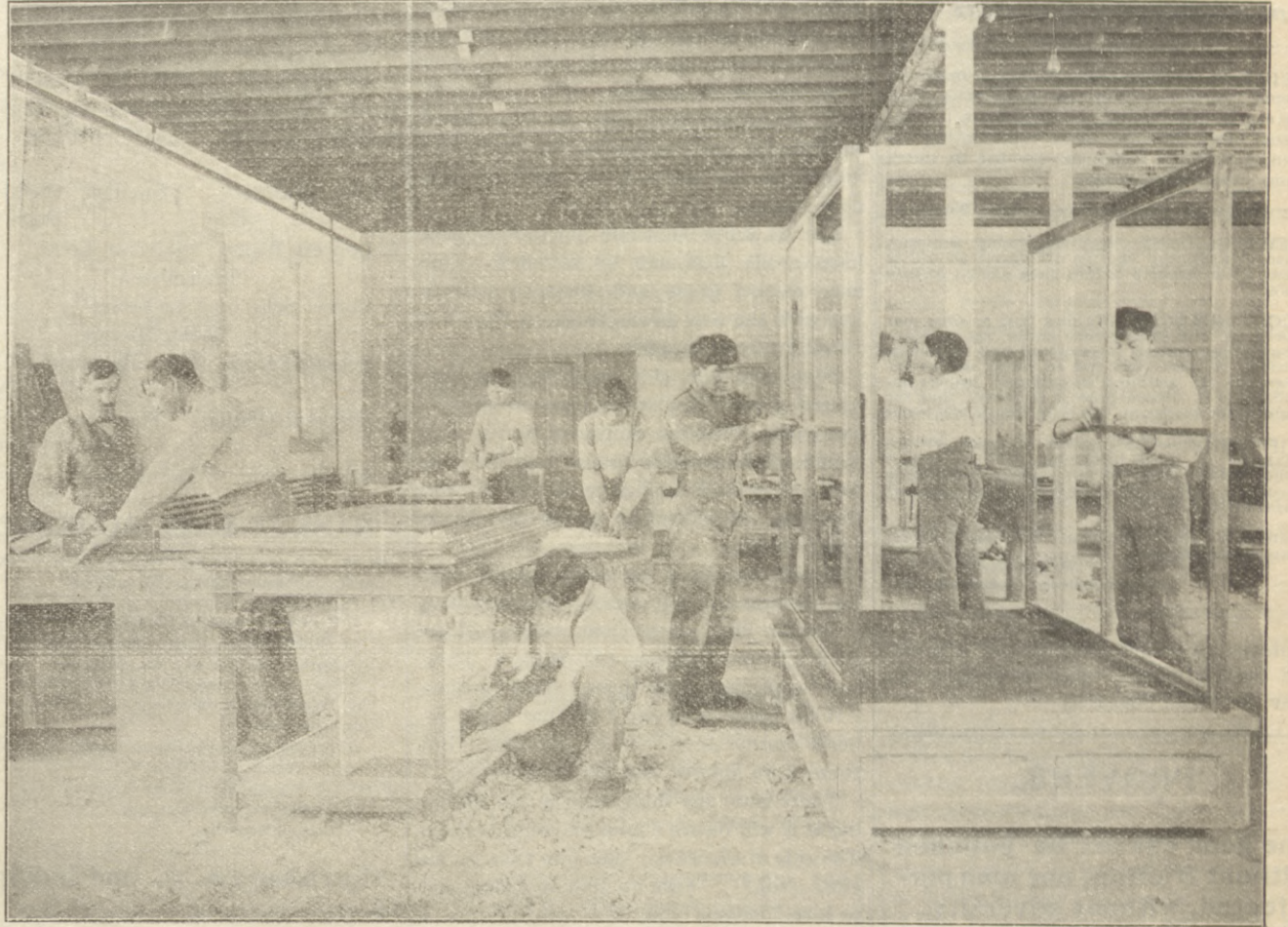
CARPENTER WORK—CABINET MAKING.
