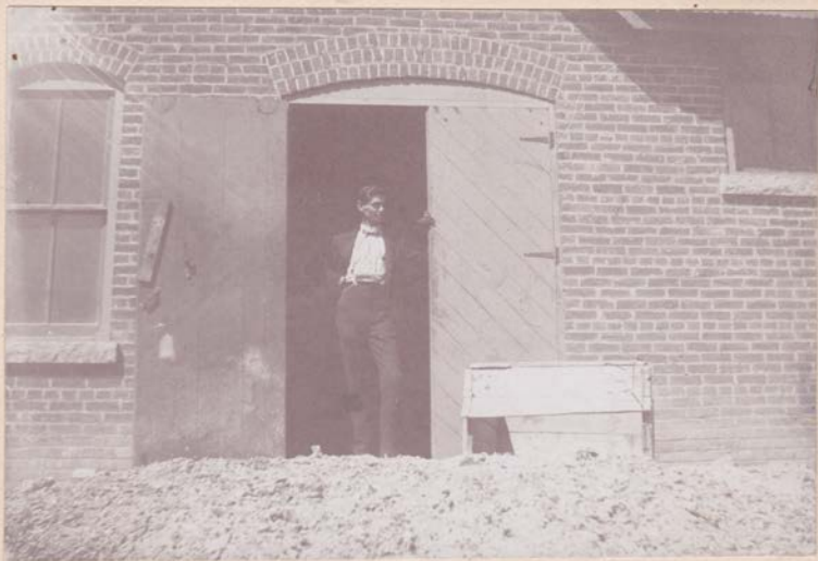
C. L. Butler Chief Engineer in Electric-lighting & steam-heating plant, with air-compressor in the rear.
